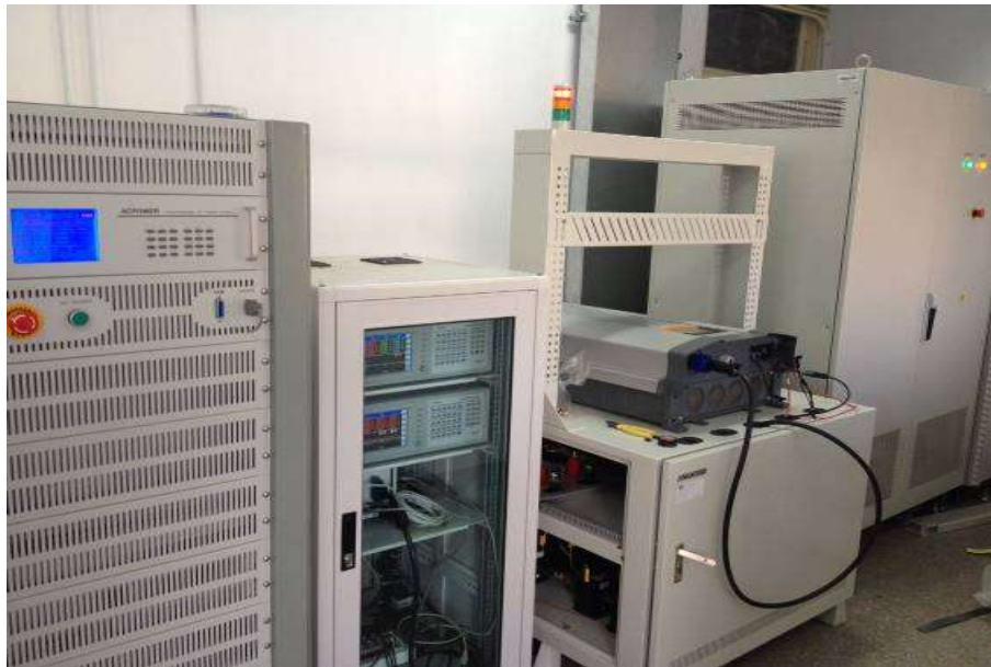
50kW PV Inverter Test System
